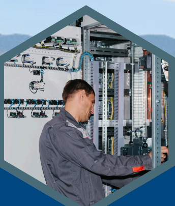
Structured Cabling & Low-Voltage Installation
