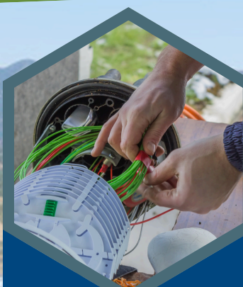
Fiber Placement & Connectivity Fit-Out
